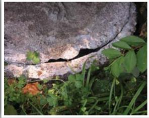
This is an example of a septic lid that is not sealed properly. Mosquitoes can easily enter through the gap.
