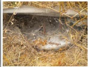
This septic is beginning to cave in and is not only a safety hazard, it allows access for mosquitoes.
