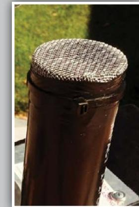
This vent pipe was screened using a fine mesh (1/16th of an inch) and secured in place using electrical tape and zip-ties.
