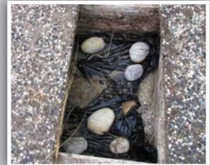
In this example the plastic does not cover the entire top of the septic. Additional sand should be used to cover the tarp as well.
