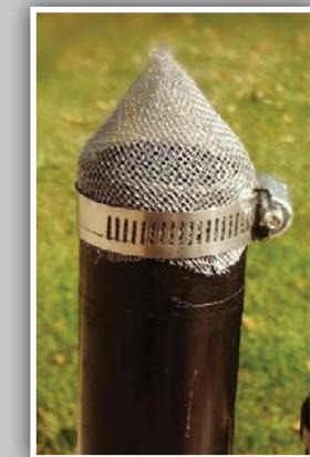
This vent pipe was screened using a fine mesh (1/16th of an inch) and secured in place with a hose clamp.
